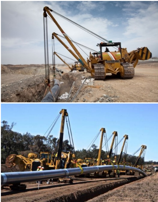
Figure 8. Trench construction and placement of pipelines on flat ground. Image source: Arabian Oil and Gas .
