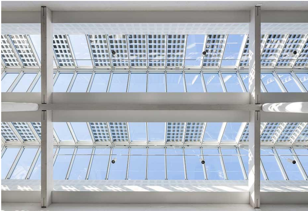
Figure 7: Building Integrated Photovoltaic Panels in the Main Lobby Skylights at Green Solution House 71
