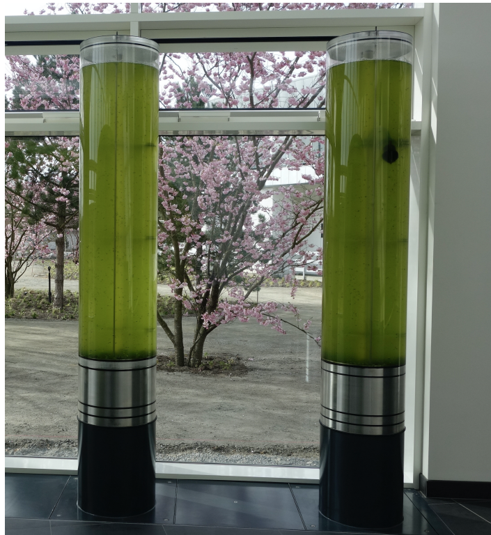
Figure 8: Algae Generators in Green Solution House's Biological Water Purification System 84
