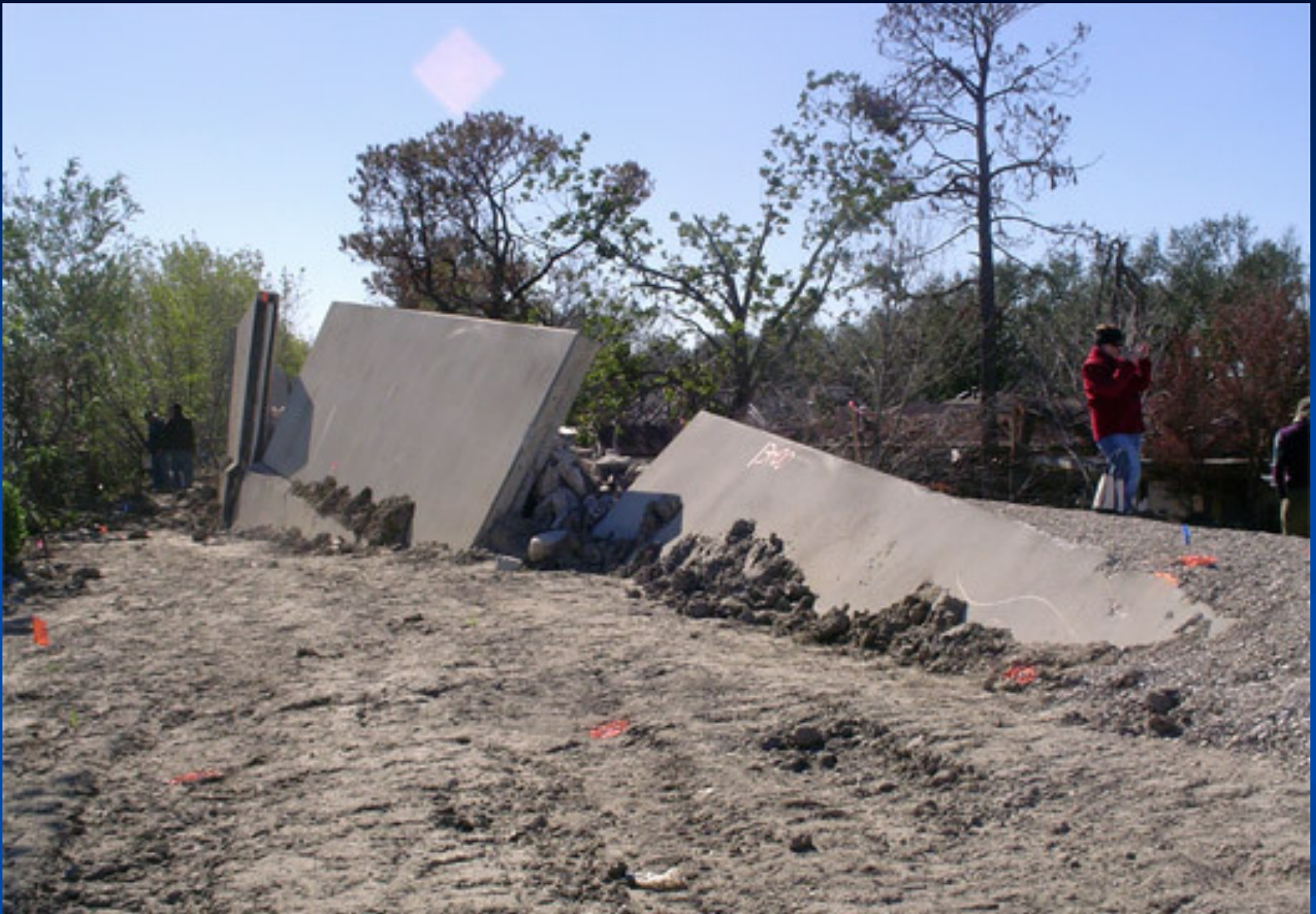
Failed floodwall and levee at 17th Street Outfall Canal, Lakeview, New Orleans, after Hurricane Katrina. [Photo by Richard Campanella]
