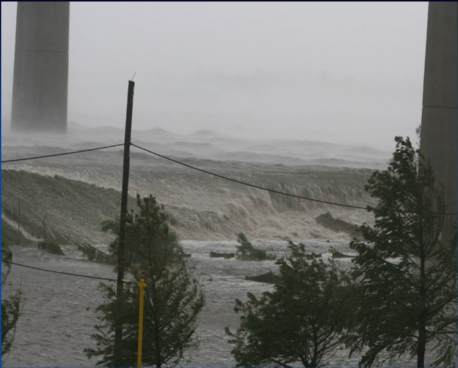
Surge tops the 8-foot high north levee of the MRGO/Intra-Coastal Canal, under the Paris Road Bridge in eastern New Orleans. Photo by Dan McClosky
