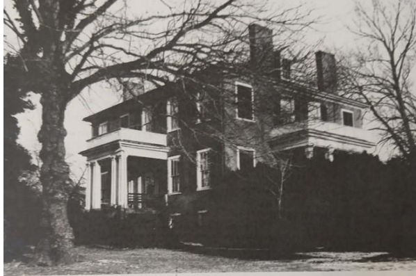
Fig 2. The Locust Grove Mansion, as seen on Page 19 in Box 57 of the Papers of K. Edward Lay, Professor of Architecture at the University of Virginia
